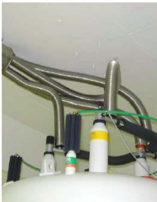
Figure 8.2: Emergency Quench Pipes
