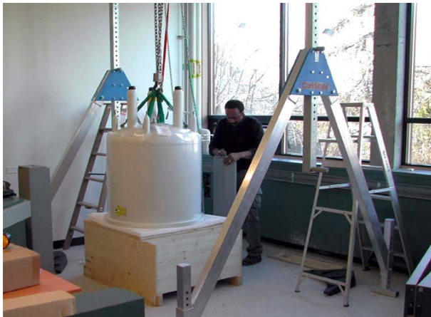
Figure 5.1: A-Frame Gantry for Lifting the Magnet Inside the Magnet Room
