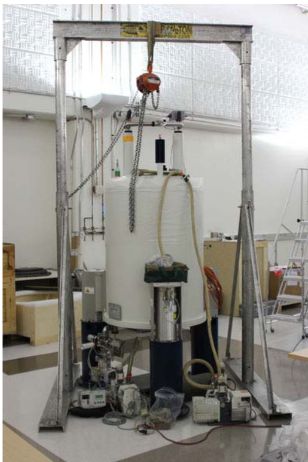
Figure 5.1: A-Frame Gantry for Lifting the Magnet Inside the Magnet Room
