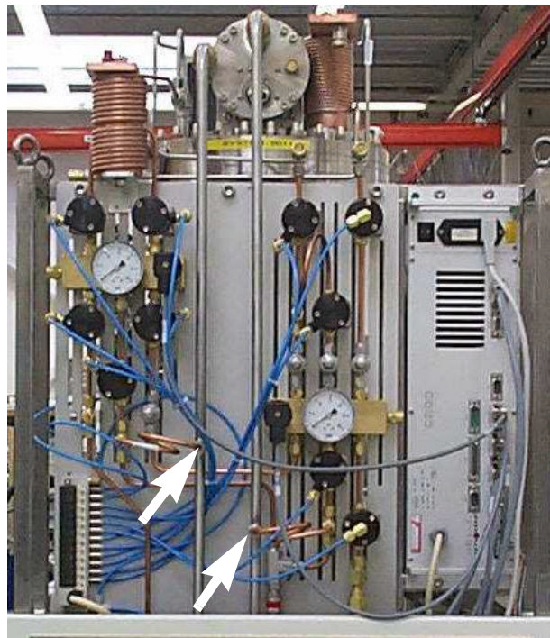
Figure 5.1. Releasing the gas from the CryoCooling Unit
