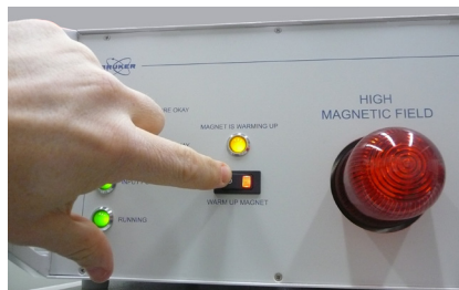
Figure 5.18: After work / service: warming up the magnet system
