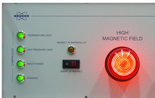
Figure 5.17: Quenching the magnet in an emergency case
