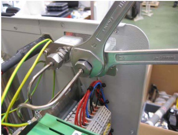
Figure 7.2: Stainless Steel Tube Removal
