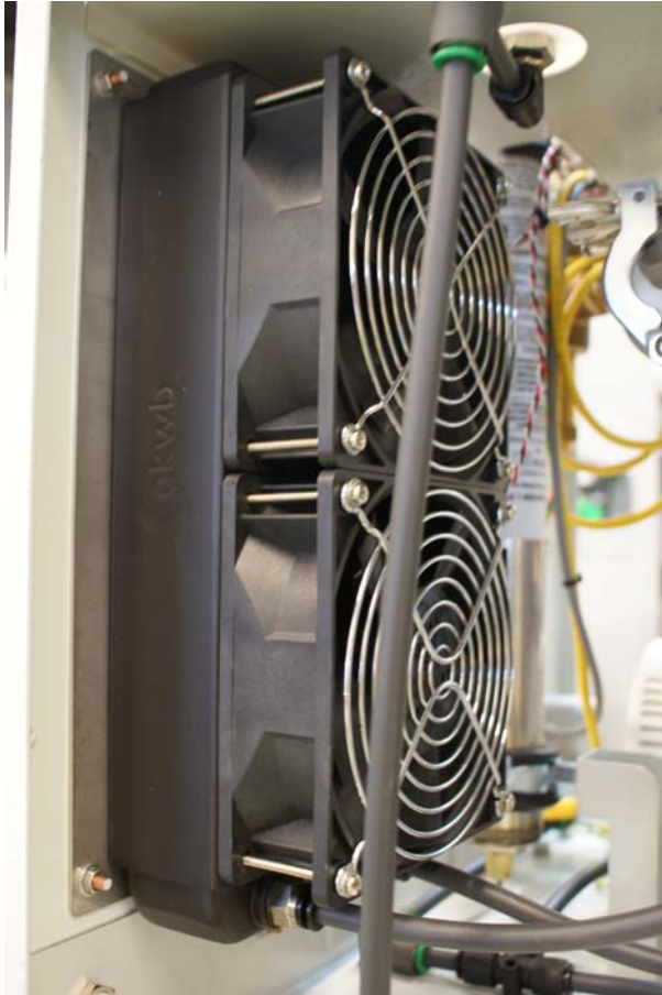
Figure 4.7: Radiator Fans
